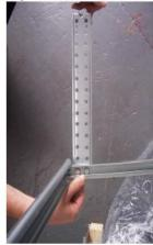
Suspend the tracks from the roof joists , they can be cut to length if required , the third track suspension plate is used as an extension piece and should be cut to length as required . When fitted you should have a gentle slope from the door end into the garage .(down hill no more than around 20mm)
