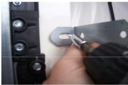
Tip! – you may find that removing the track either side by undoing the bolt that holds the track to the frame makes it easier to obtain a good fixing point.
