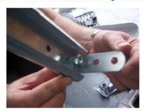
GARAGEDOORSONLINE www.garagedoorsonline.co.uk 01926 463888 Attach the rear track suspension bar (Located at the top of the frame on the inside when delivered ) then attach the track
