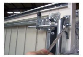
Now bolt the brackets to the wall with 50mm coach screws you will need Rawl plugs (not supplied) at this stage . Ensure the brackets are firmly fixed in place and the door is rigid .
